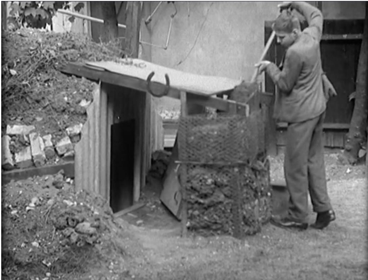
Joonis 1 Andersoni punkri ehitamine, https://andersonshelters.org.uk/design-construction/building/
