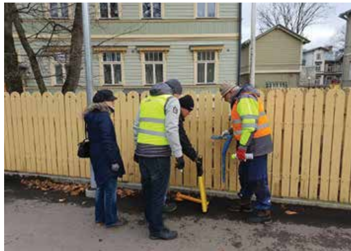
Picture 25: Detecting street lighting cables with EML in Vesivärava Street
