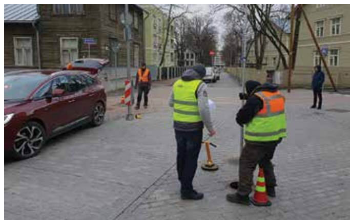
Picture 28: Inspection of the sewerage manholes in Vesivärava Street
