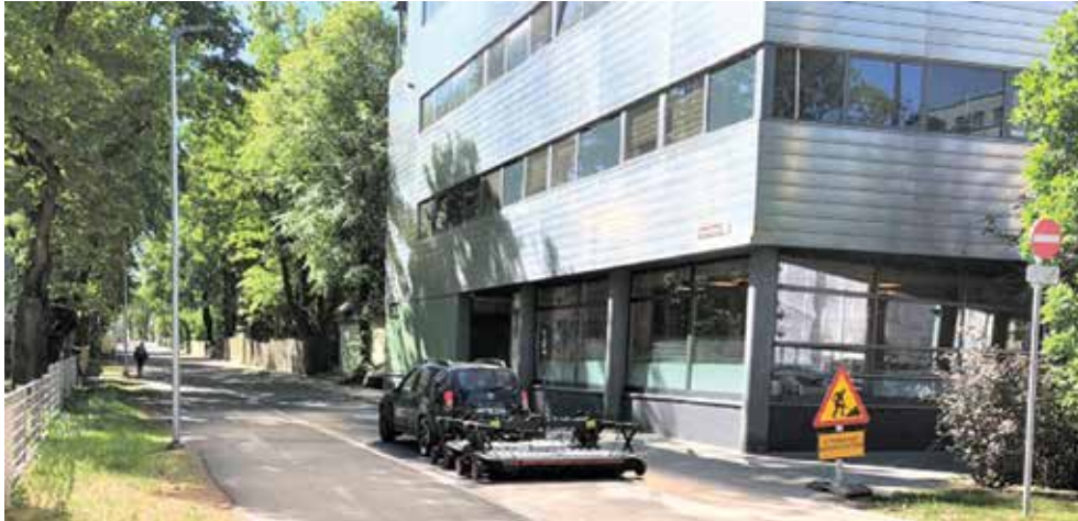
Picture 13: View of Vesivärava Street from Raua Street with IDS Stream EM GPR
