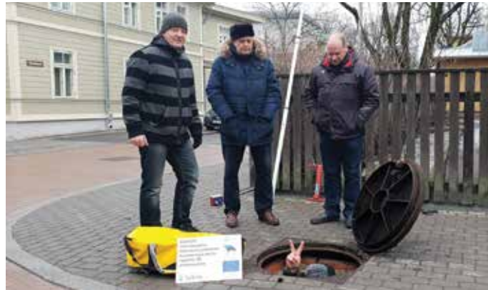
Picture 27: Inspection of telecom manhole in Vesivärava Street
