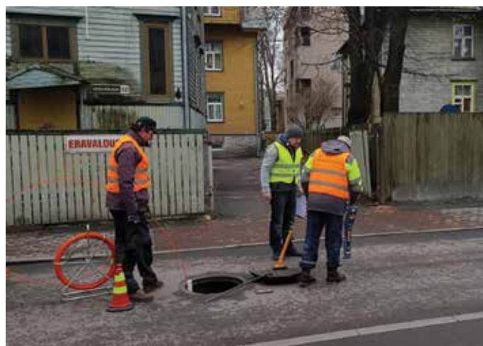
Picture 26: Measuring stormwater sewerage with a sonde in Vesivärava Street
